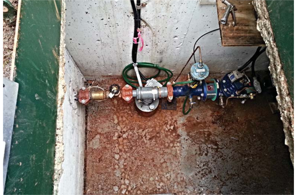
Well #4 - Wellhead completion
