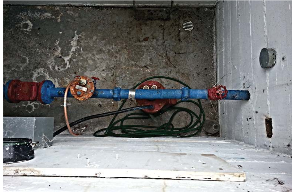
Well #2 - Wellhead completion
