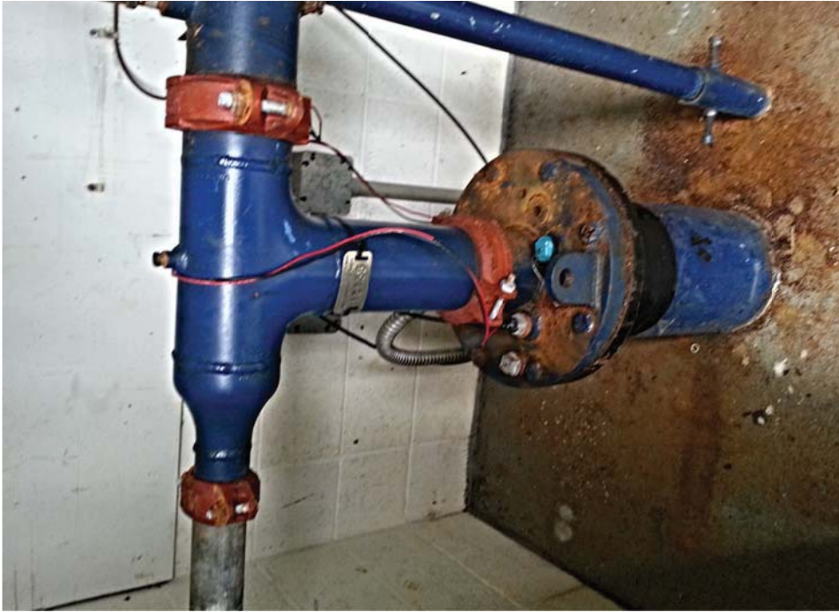
Well #5 - Wellhead Completion
