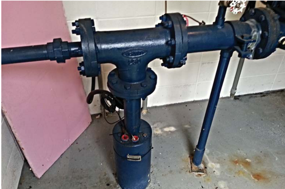
Well #6 - Wellhead completion
