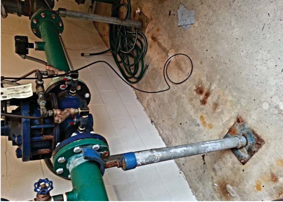
Well #8 - Wellhead Completion
