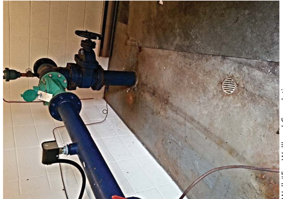
Well #5 - Wellhead Completion
