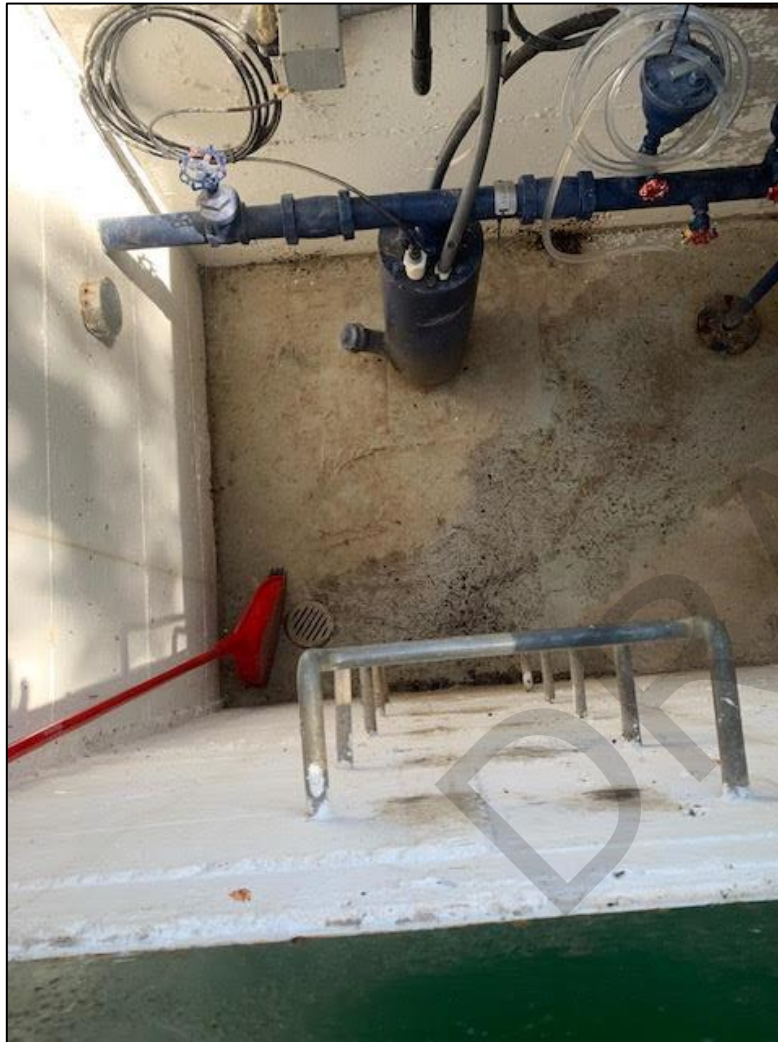
Photograph B3 (LEFT): Looking down into the well pit floor, floor drain and the top of the wellhead for Well 1. Photograph B4 (RIGHT): Close up view of the well head for Well 1. Visible is the intact concrete floor around the well casing, the well connected to the water distribution system, the electrical line for the well pump and the connection for the pressure transducer.
