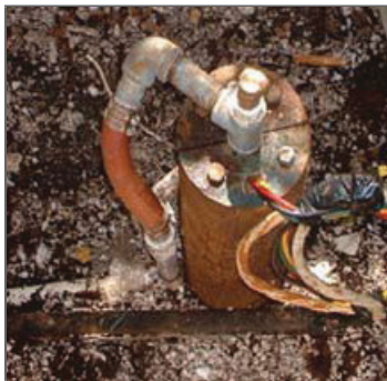
FIGURE 5 Well with sanitary seal type cap
