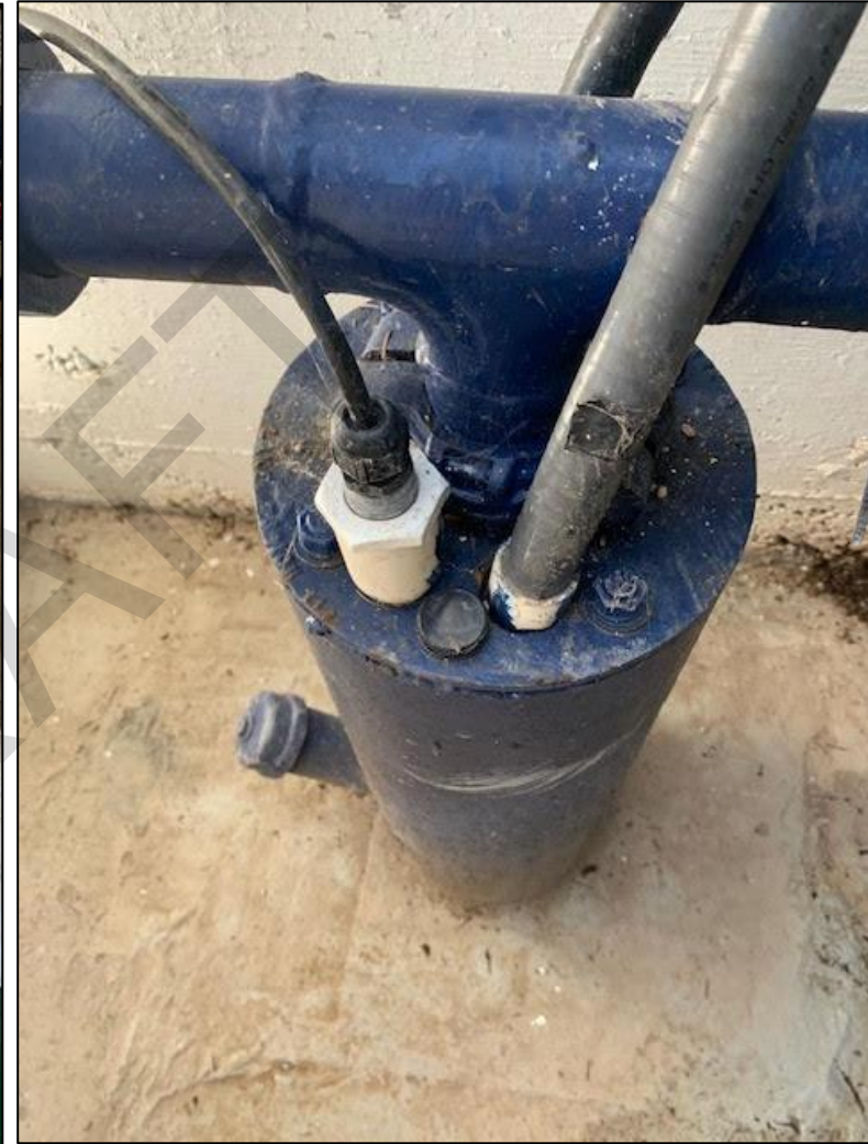
Photograph B3 (LEFT): Looking down into the well pit floor, floor drain and the top of the wellhead for Well 1. Photograph B4 (RIGHT): Close up view of the well head for Well 1. Visible is the intact concrete floor around the well casing, the well connected to the water distribution system, the electrical line for the well pump and the connection for the pressure transducer.
