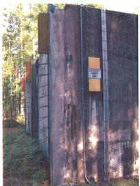
The defects also coincide with what appears to be previous concrete repair work. It is understood from the board that there is some record of these repairs being carried out in around 2001.
