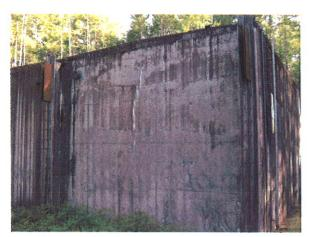
The general concrete surface of the tank appears in reasonable condition. There are some cracks which are leeching salts which are midspan of the tank and may require repair.
