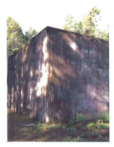
No spalling could be seen and the significant defects appear confined to the corners of the tank. It is understood that these defects are not evident on the inside of the tank; however it is recommended that a review of the interior be made to confirm this as it may help define the appropriate repair strategy.
